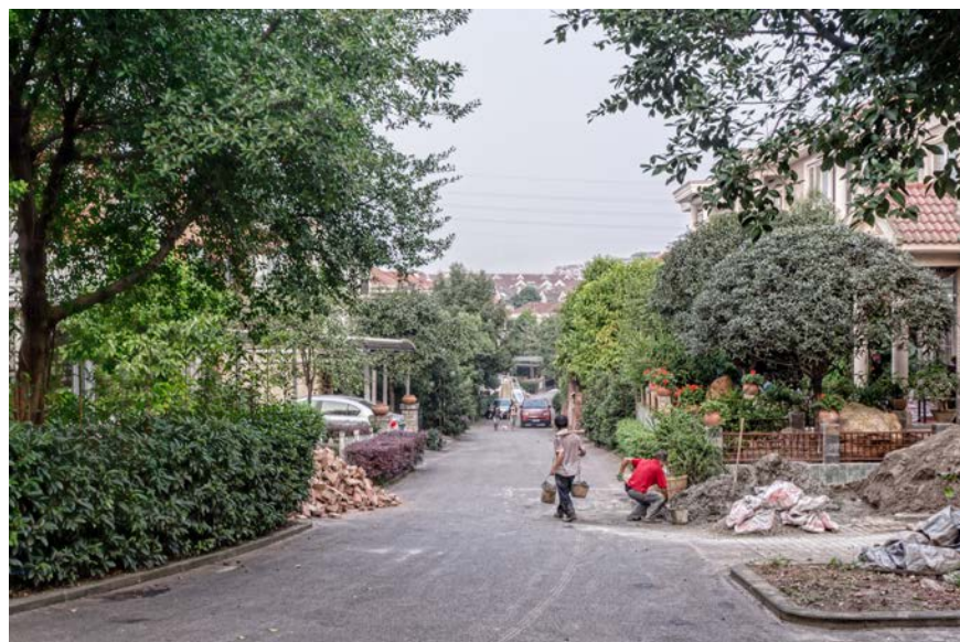
Figure 17 Workers mixing and carrying concrete to side of house
