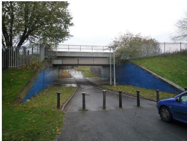
Bridge on Taylor Street after painting with anti-graffiti paint
