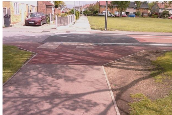
Route AFTER removal of street clutter
