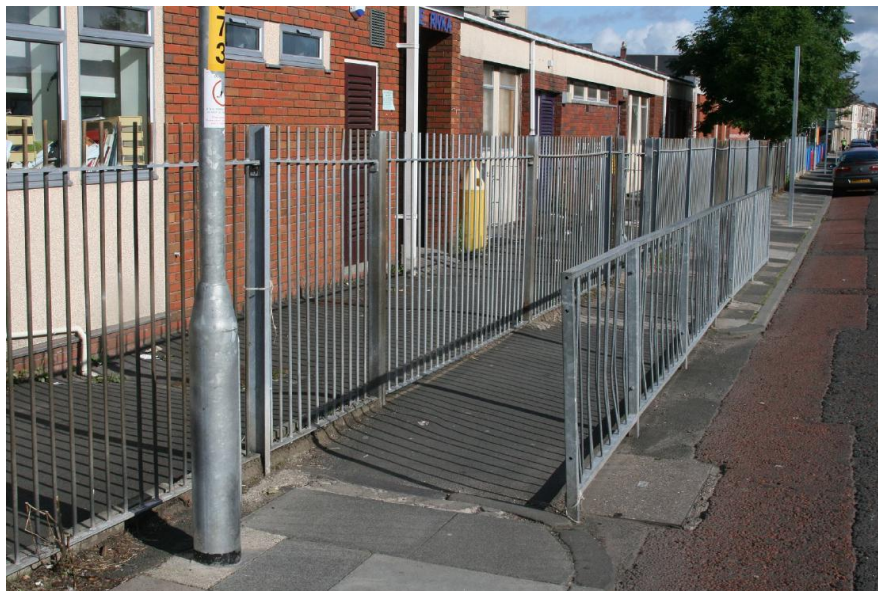
Guard rail prior to FFW intervention
