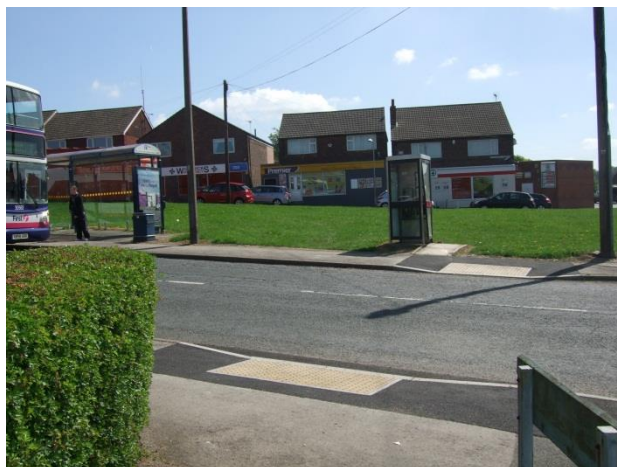
New dropped kerb crossing on Addison Road
