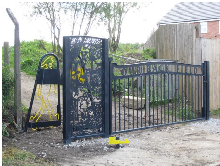
Entrance to the field AFTER new gate installed
