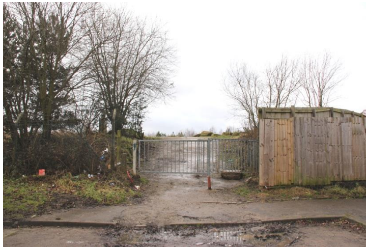
Entrance to the field BEFORE new gate installed
