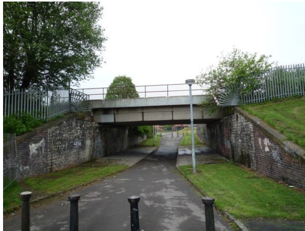
Bridge on Taylor Street before improvements
