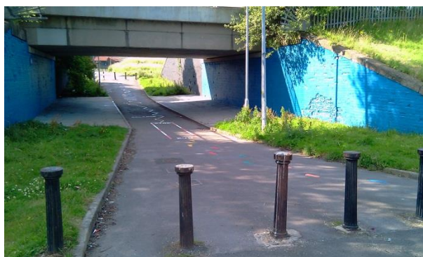
New footsteps marked on pavement under bridge
