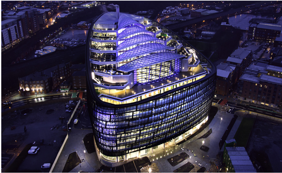
Figure 4.6: Case-study building (BuroHappold Engineering and Palin, 2016)
