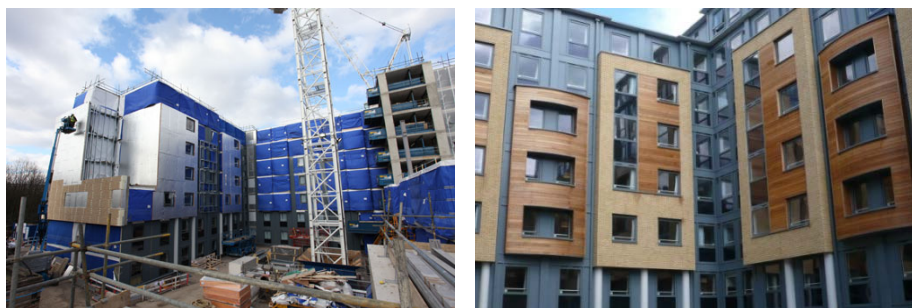
Figure 4.1 (left): [REDACTED] building during construction [REDACTED] 2012]
