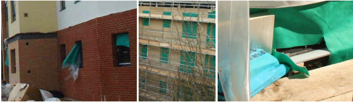
Figure 7.58 (left): Breather membranes still visible after cladding construction [REDACTED] 2012]
