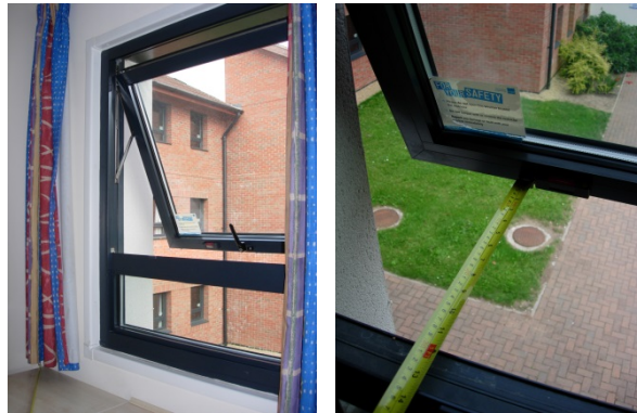
Figure 5.18 (left): Loughborough study – Extent of modular window opening Figure 5.19 (centre): Loughborough study – Modular windows fully open at 30cm
