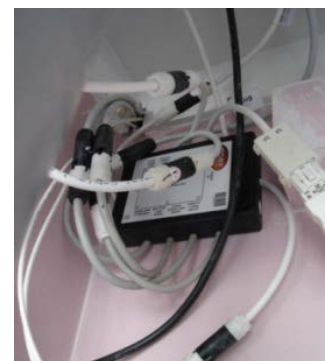
Figure 4.19: Modular wiring system
