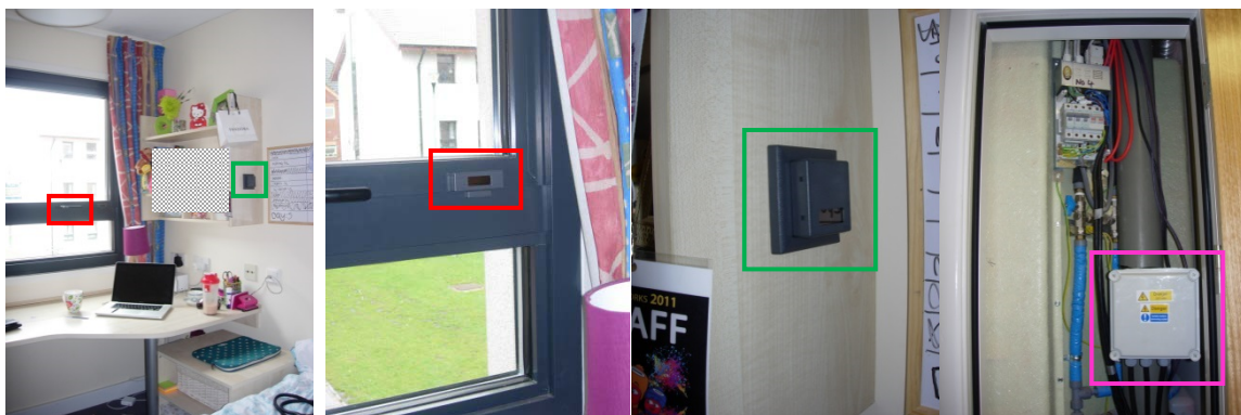
Figure C.10 (far left): Temperature sensor and window contact installed for pilot study
