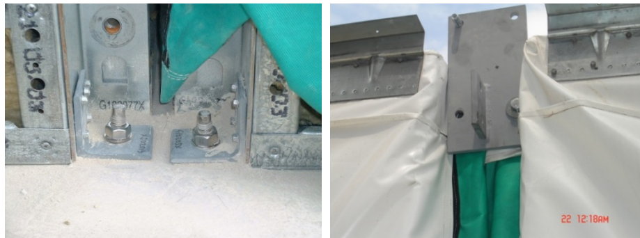
Figure F.1 (left): Two adjacent modules fitted to the foundations [REDACTED] 2012]
