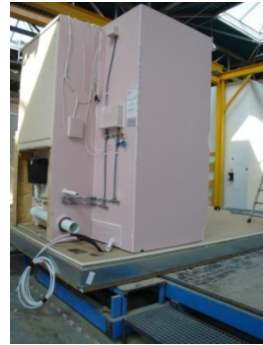
Figure H.12 (left): Shower pod ready to be lifted onto floor panel
