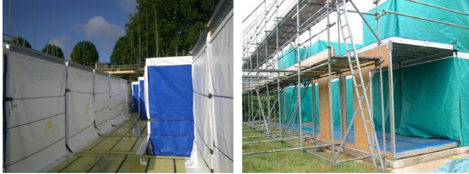
Figure 4.16 (left): Corridor onstruction on site – floor cassettes fitted between modules [REDACTED] 2012]
