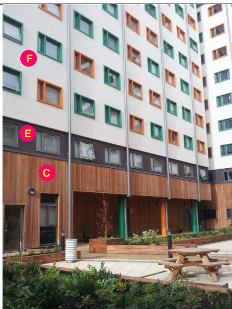
Block B East facing facade facing the courtyard
