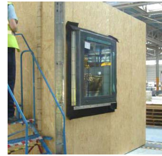
Figure 5.48: Window fitted to external face of module in factory
