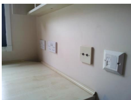
Figure 7.4 (left): Air leakage path through sockets in modules: Loughborough case study
