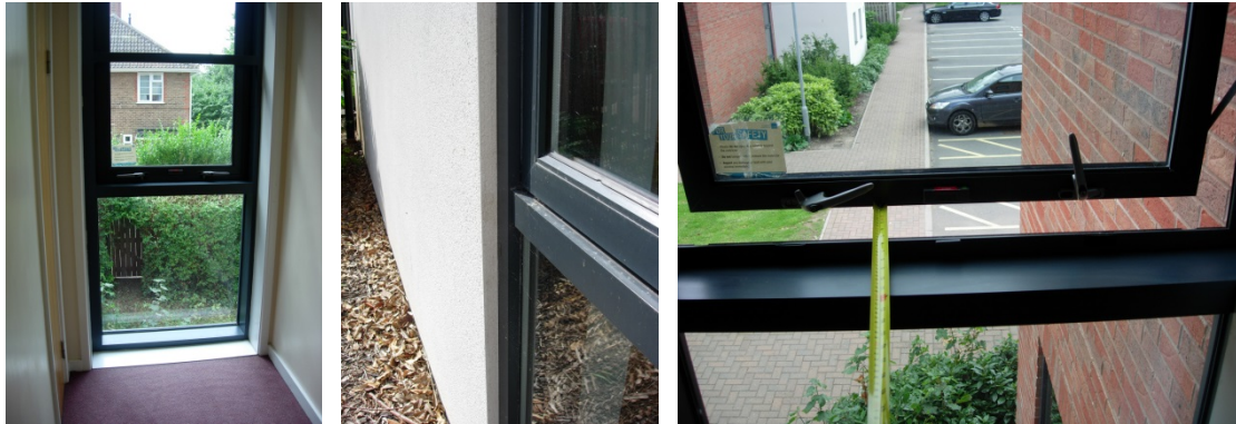
Figure 5.20 (left): Loughborough study: curtain walling within student flat
