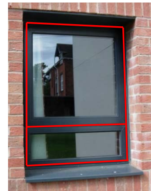
Figure 7.39: Greatest heat losses at thinnest part of frames – marked red
