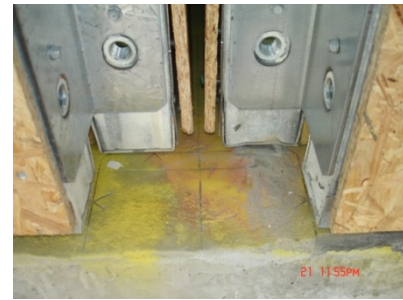
Figure 7.14: Air gap at party wall junction between modules [REDACTED] 2012]
