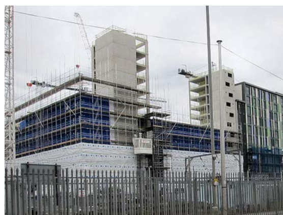
Figure 5.40 : London study – Block B non-modular cores completed and modules partly installed [REDACTED], 2014]
