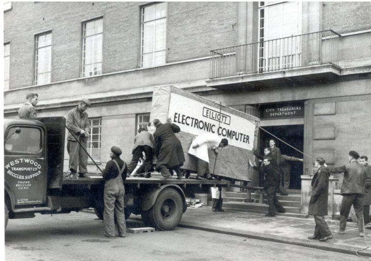
Figure 1: Elliot 405 Computer Delivered at Norwich City Council, 1957
