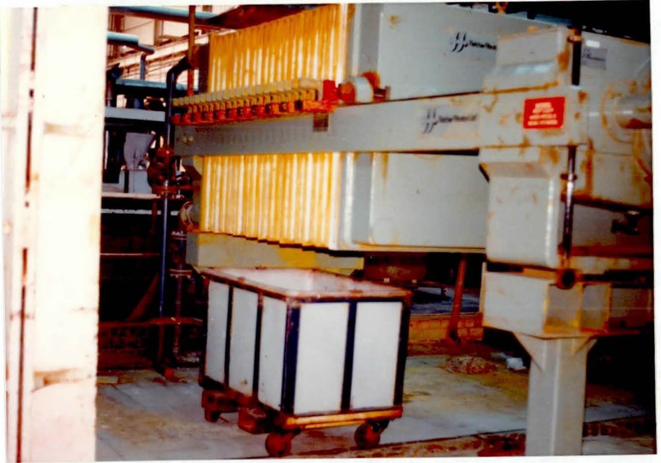
FIG 4-1 FILTER PRESS WITH A SKIP UNDER THE PACK
