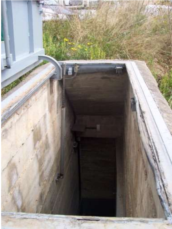
Figure 2.4 Entrance to a utility tunnel in Barcelona. Source: Canto-Perello et al. (2009)
