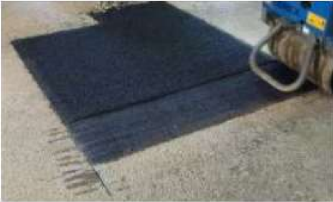
Figure 2.2 Temporary backfilled pavement. Source: Department for Transport (2014)
