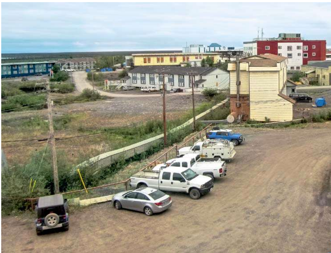
Figure 2.6 An over-ground Utilidor running along the edge of a car park in Inuvik. (Source: Herrington, 2013)
