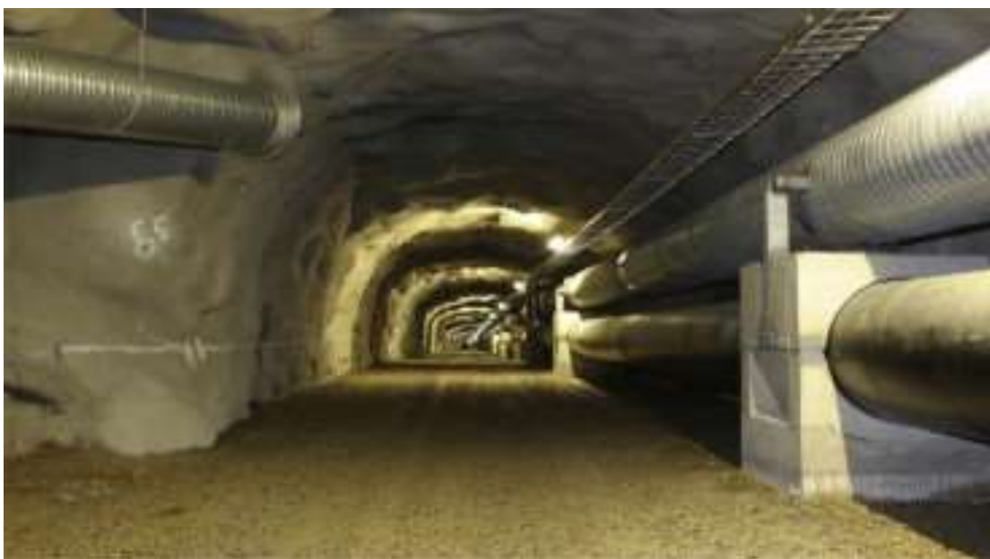
Figure 2.5 A typical utility tunnel in Helsinki. Source: Vahaaho (2014)
