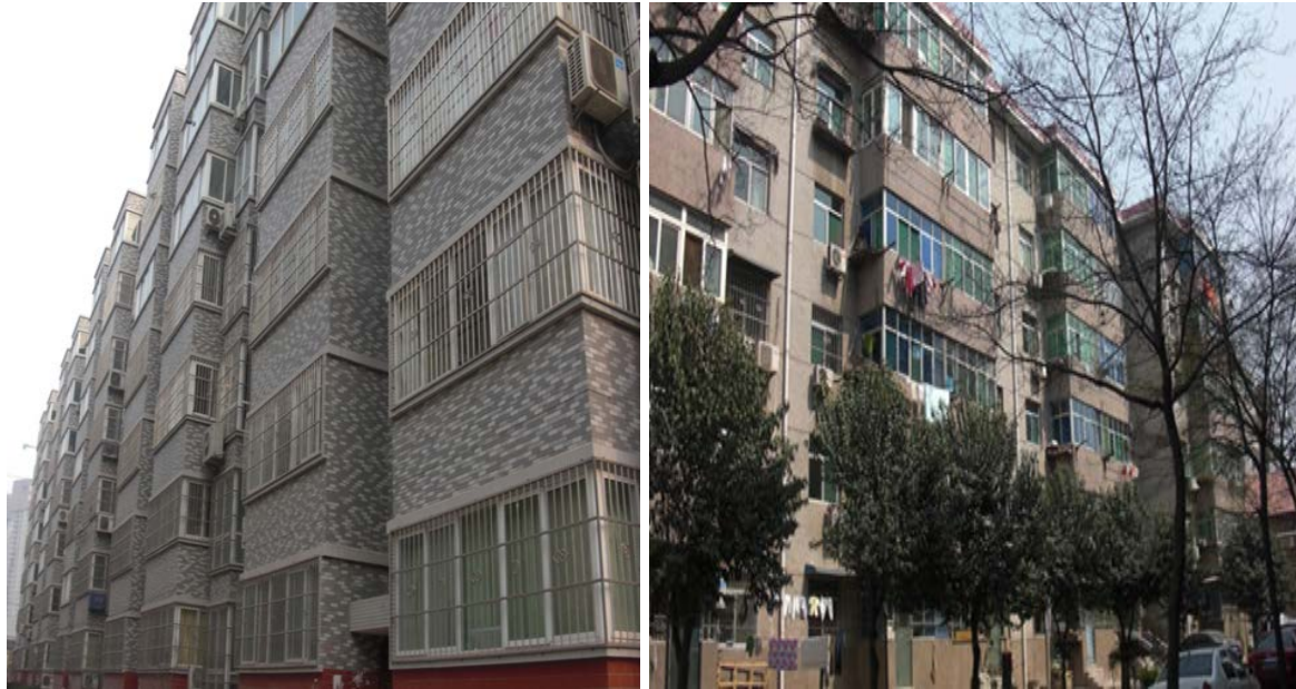
Figure 3.2(a) the typical investigated new building; (b) the typical investigated old building
