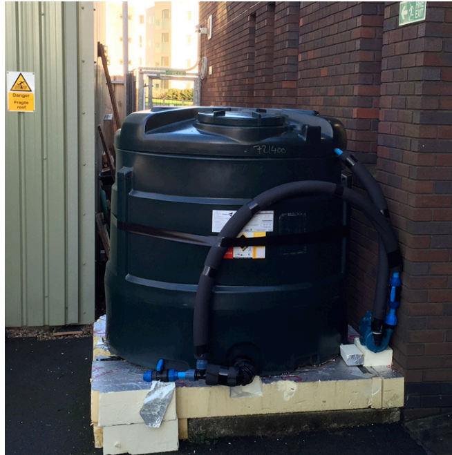
Photograph 1. Oil tank adapted for use as biogas reactor for food waste processing
