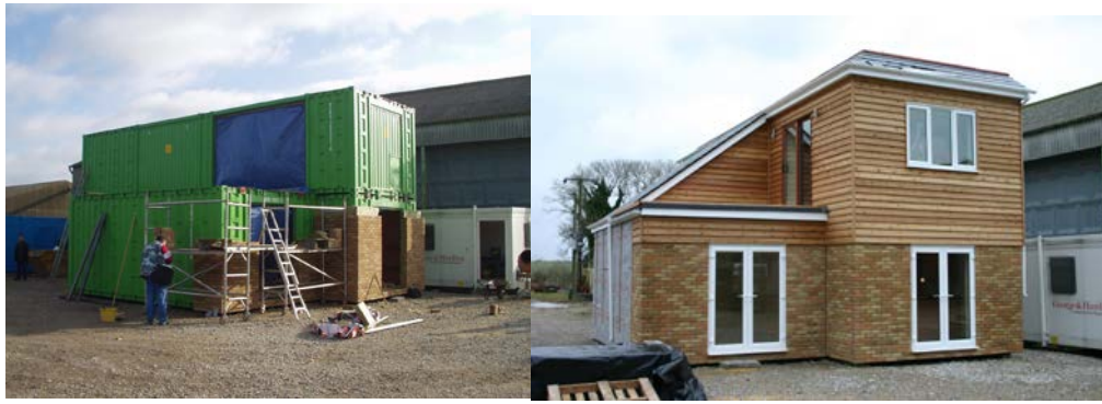
Figure 4.12 Assembly and completion of prototype house at Broxbourne, UK (source: Verbus)
