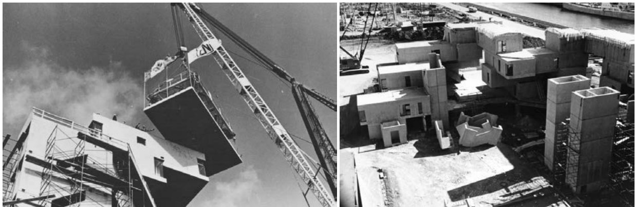
Figure 1.2 & 1.3 Precast modular construction for Habitat'67 (source: Moshe Safdie archive www.habitat67.com )
