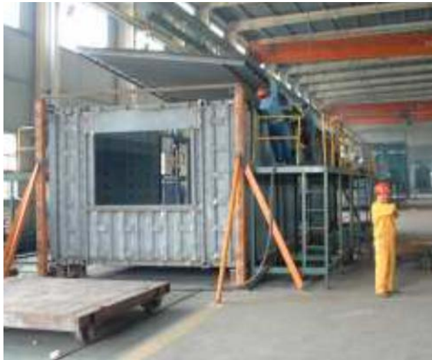
Figure 4.42 Production of first run of containers for multi-storey construction
