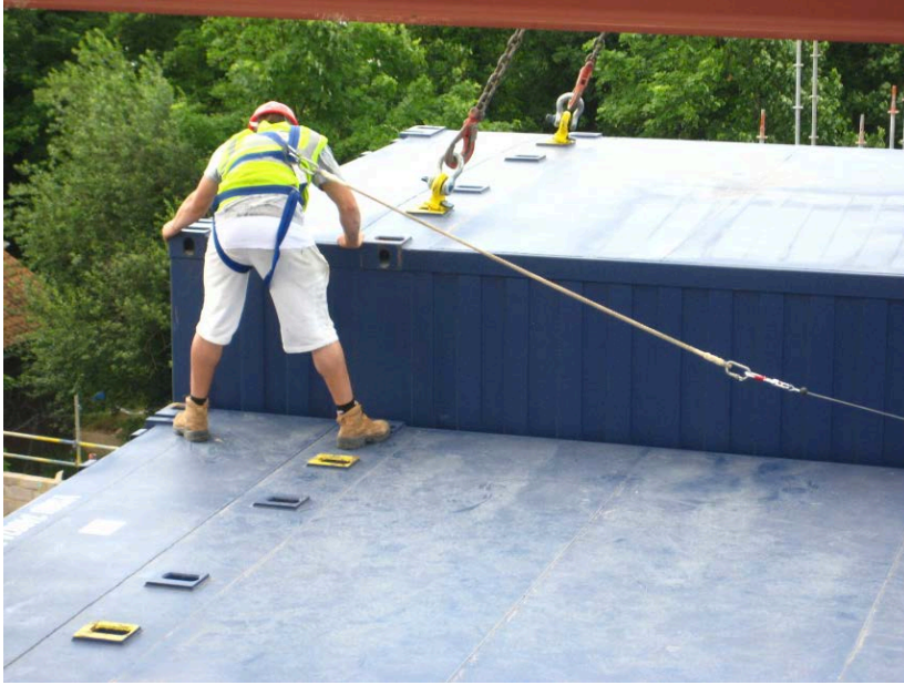
Figure 4.24 Lowering of units guided by site installers wearing man-safes (source: author)
