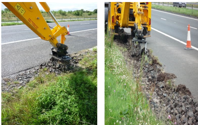
Figure 5 Scarifying exercise on the M77/GSO DBFOs.
