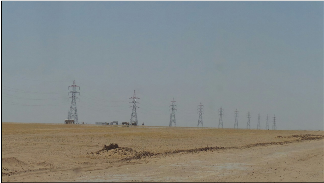
Figure 5.7 Electrical tower to connect electricity from Shagaya farm to the main station
