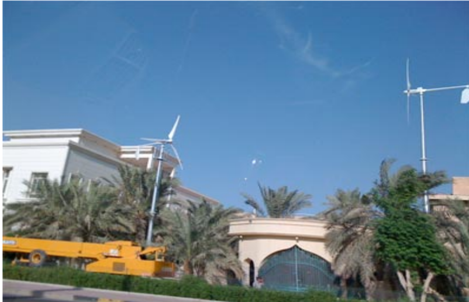
Figure 8.3 A house in Kuwait using wind turbine to generate energy for the house
