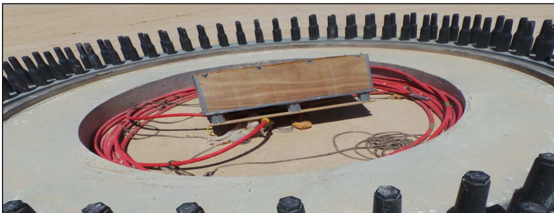
Figure 5.5 Electrical work for wind turbine tower connection
