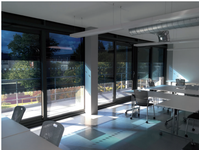
Figure 1 Example Sage Glass electrochromic glazing installation (Architecture Building, Loughborough University, UK)
