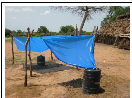
Photograph 1. Example of Plastic Sheet Rainwater Harvesting Systems
