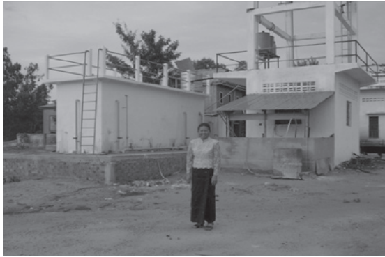
Picture 3. Mrs Meas Yan in front of her treatment plant
