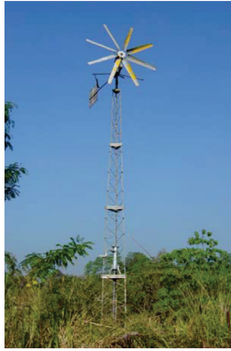
Figure 6. Pilot wind pump assembly
