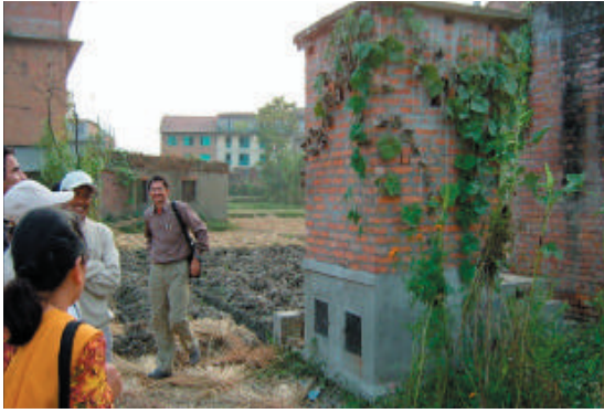
Photograph 3. ECOSAN toilet in use
