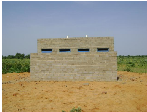
Figure 1. Latrine constructed with SSBs
