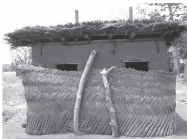
Photograph 1. VIP built with local materials
