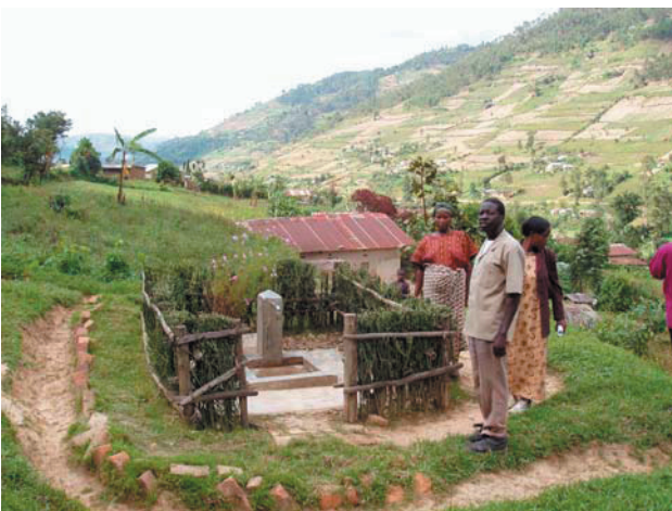
Photograph 3. A public tapstand in a gravity flow scheme
