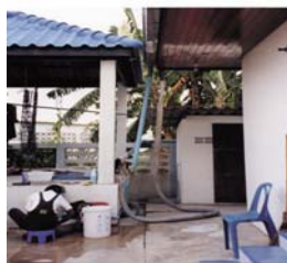
Figure 2. Household collects rainwater from rooftop and stores in a tank built on the ground
