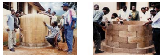
Figure 7. Training on construction of rainwater jar and tank in Tanzania
