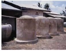
Figure 4. Household collects rainwater in a series of four tanks
