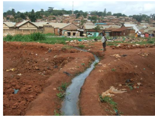
Photograph 2. Septic tank effluent channelled down to soakaway near spring
