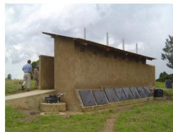
Photograph 2 - Rear view showing access panels
