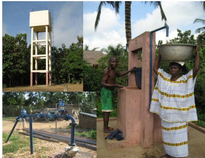
Photograph 1. Components of a piped network. Clockwise from bottom left: borehole; water tower; and standpost with water seller and user
