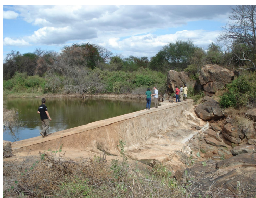
Photograph 1. partly full dam
