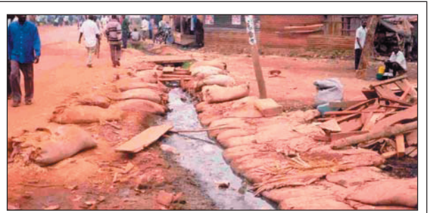
Photograph 10. Using sand bags to divert surface flows
