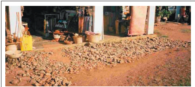
Photograph 6. A pervious pavement
