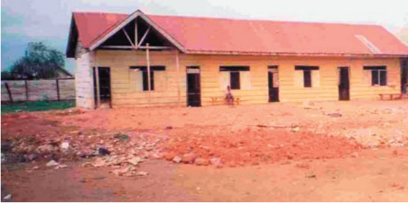
Photograph 11. Raising the ground level to avoid flooding
