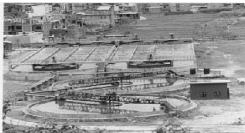
Figure 2. Oxidation ditch and secondary clarifier
