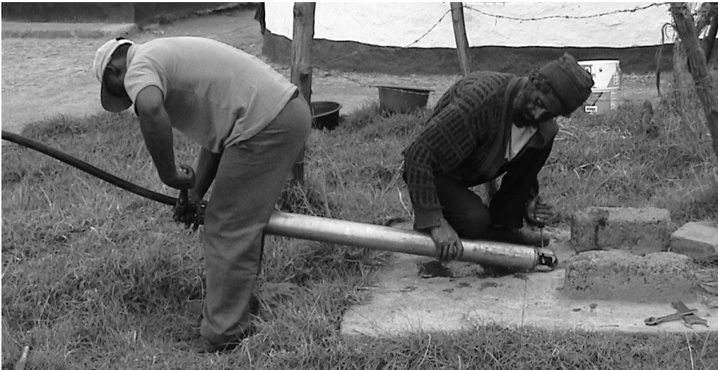
Photograph 7.2. APM undertaking Vergnet pump repairs
