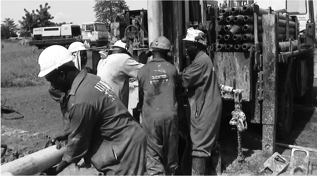
Photograph 6.3. Installing uPVC casing and screening in a newly drilled borehole
