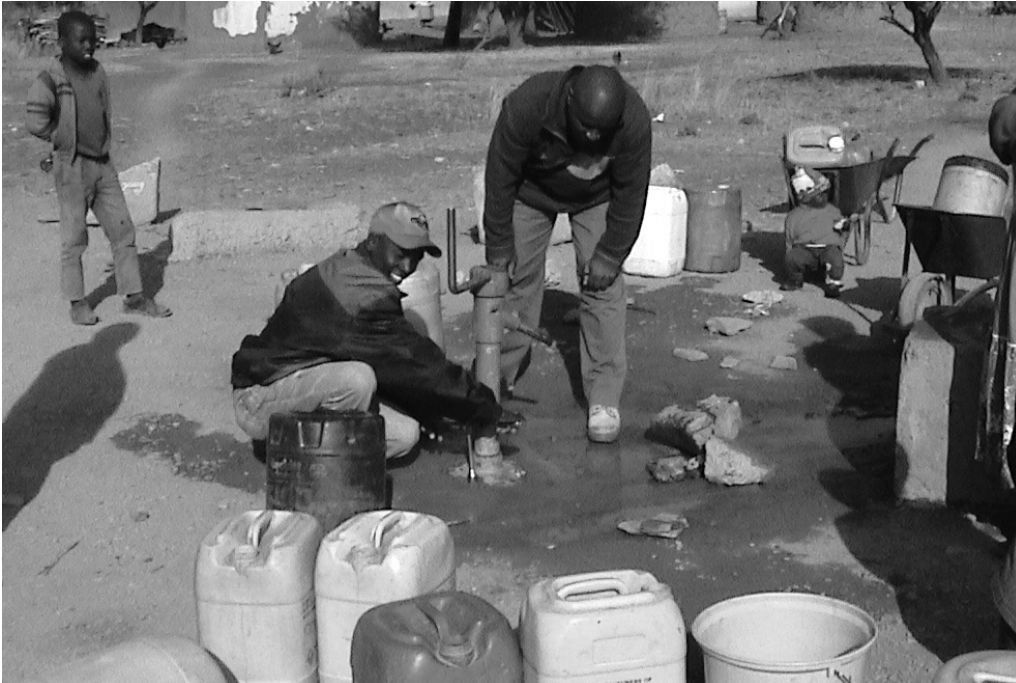
Photograph 7.3. Contractor undertaking maintenance on a Mono pump in South Africa
