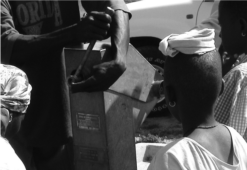
Photograph 7.1. Volunteer removing Afridev pump cover for routine maintenance
