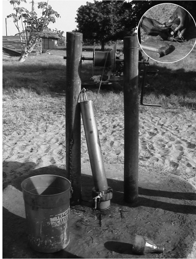
Photograph 6.7. Bucket pump on tubewell, and undergoing repair
