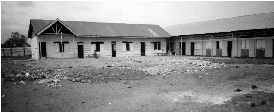
Figure 6.23. This school is being built on raised ground to avoid the frequent floods in the area
