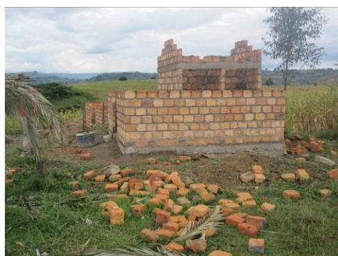
Latrines and washrooms under construction
