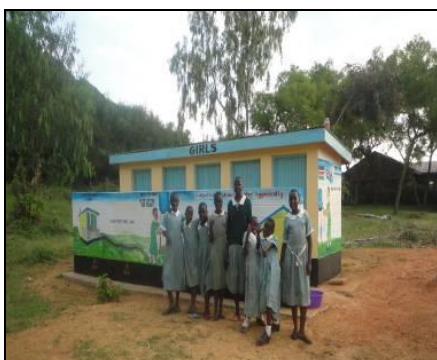
Photograph 2. Girls latrine after intervention
