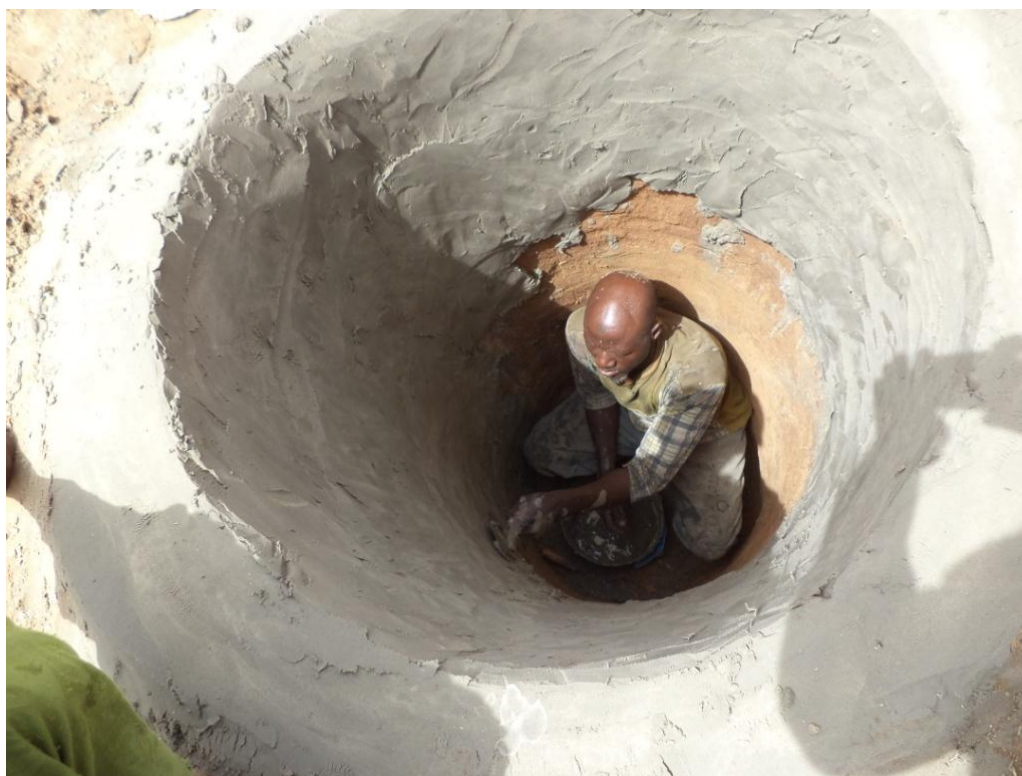
Photograph 8. Latrine walls rendered with cement to stabilise walls
