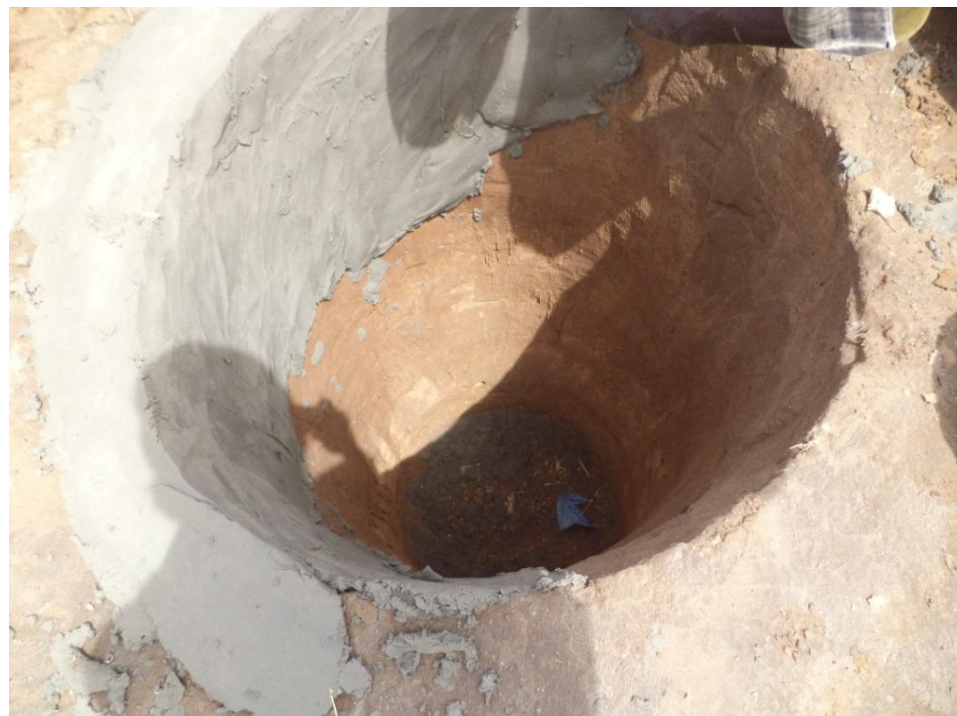
Photograph 7. Latrine walls rendered with cement to stabilise walls
