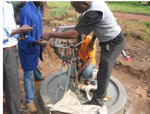
Photograph 4. Installing Rope Pump during training (Squatting is the Drilling trainer).
