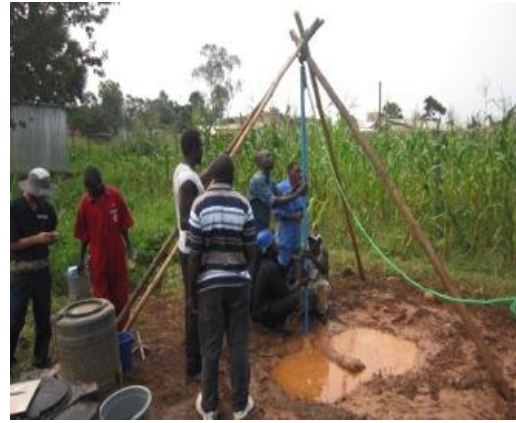
Photograph 2. Trainees drilling their very first well of 22m deep during training
