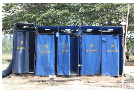
Photograph 1. Toilets provided by Public Works installed in Tiganderket
