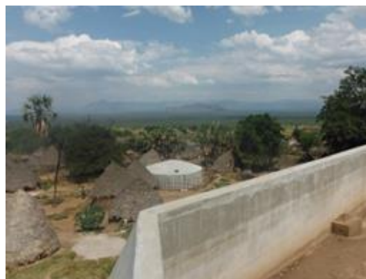
Photograph 2. Completed rock catchment system in Mohina. View from the weir.
