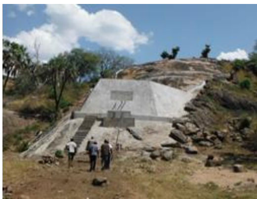
Photograph 1. Completed rock catchment system in Mohina. View from the tank.
