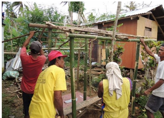
Photo 1. Community construction of a Rapid Response latrine
