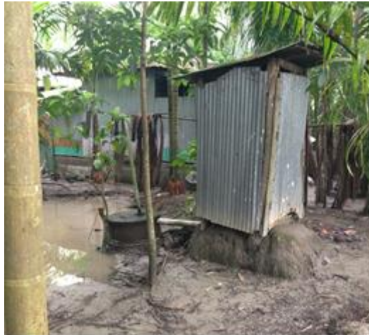
Photograph 1. Latrines that leak faeces
