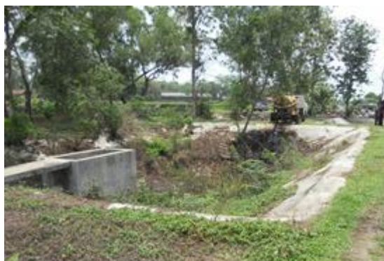
Photograph 1. Underloaded Metro anaerobic pond
