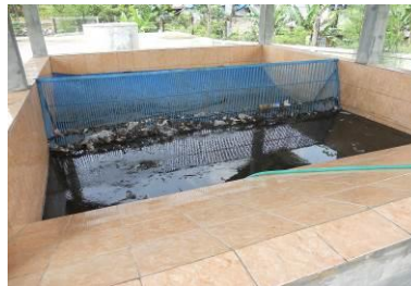
Photograph 3. Vertical screen with no operator access
