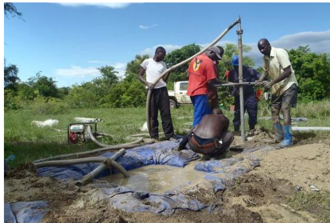
Photograph 1. Rotary well jetting in developmental context 3
