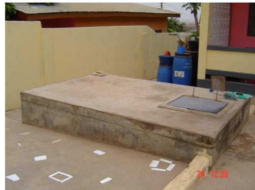
Photograph 2. Water storage facilities
