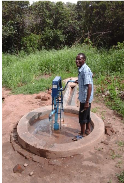
Figure 1. Communal Rope pump installed on an existing hand dug
