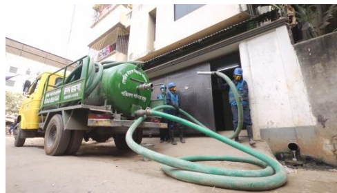
Photograph 5. MSEs emptying septic tank
