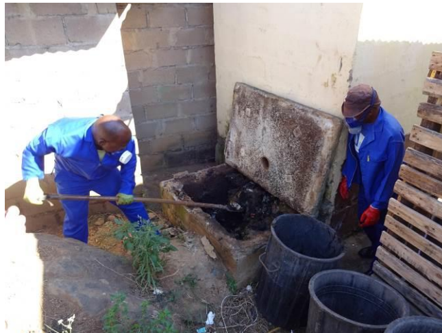
Photograph 5. Manual emptying of dry pits with trash in Durban, South Africa
