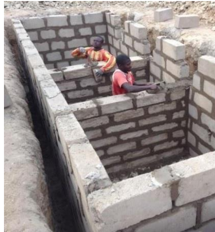
Photograph 2. CRS Ghana – pit of school latrine under construction
