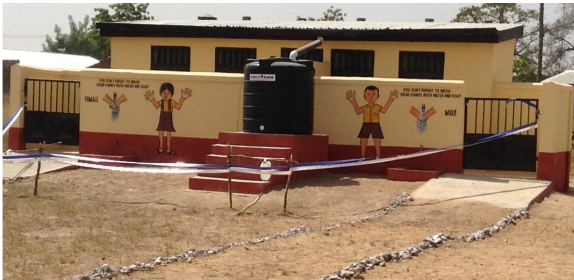
Photograph 3. CRS – a completed school latrine with WASH murals
