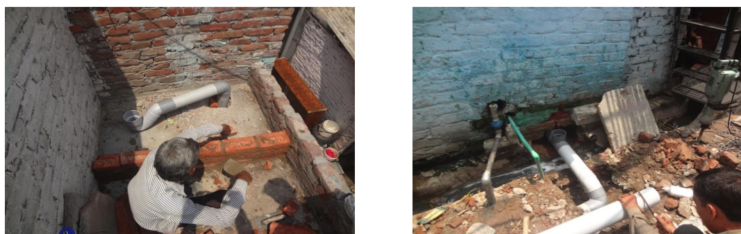
Photograph 4: Household toilet being constructed & connected with simplified sewer line
