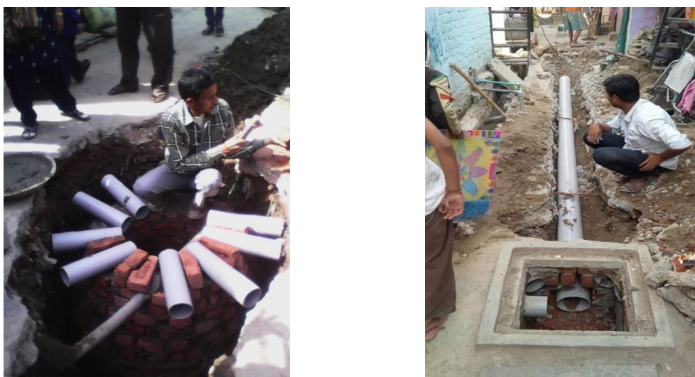
Photograph 3. Simplified sewer line being laid at Safeda Basti
