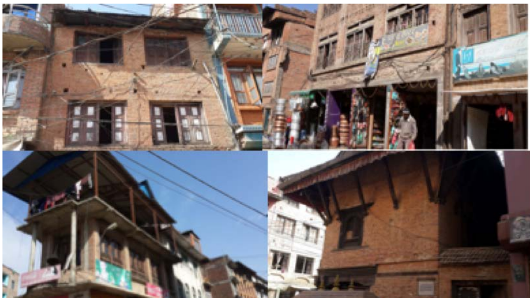
Figure 1 Examples of building types: Load bearing wall building with plank wooden floor and CGI roof; Timber frame on the ground floor and Load bearing brick wall on an upper floor; RCC frame Masonry Infill wall building with Steel Skeleton on the top floor; Partly Load Bearing Wall and Partly timber column (authors' pictures)
