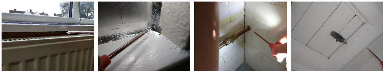
Figure 7 - Qualitative air leakage testing using smoke sticks
