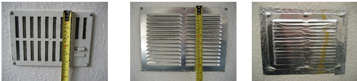
Figure 5 - Fireplace vents sealed with aluminium tape to ensure uniformity between houses
