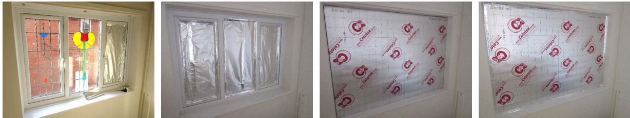
Figure 4 - Application of foil and insulation to landing windows to reduce east/west solar gain
