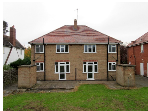
Figure 2 – Loughborough matched pair test Houses viewed from the rear
