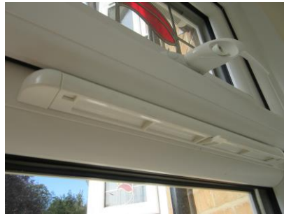
Figure 3 – Trickle vent closed
