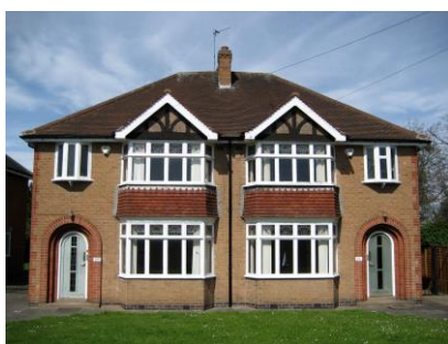
Figure 1 – Ashby Road Test Houses pre-refurbishment, only the left house was used
