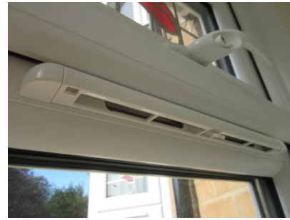
Figure 4 – Trickle vent open
