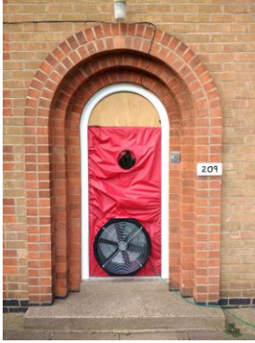
Figure 6 – Front door with a semi-circular wooden panel to fill the gap in the upper arch.
