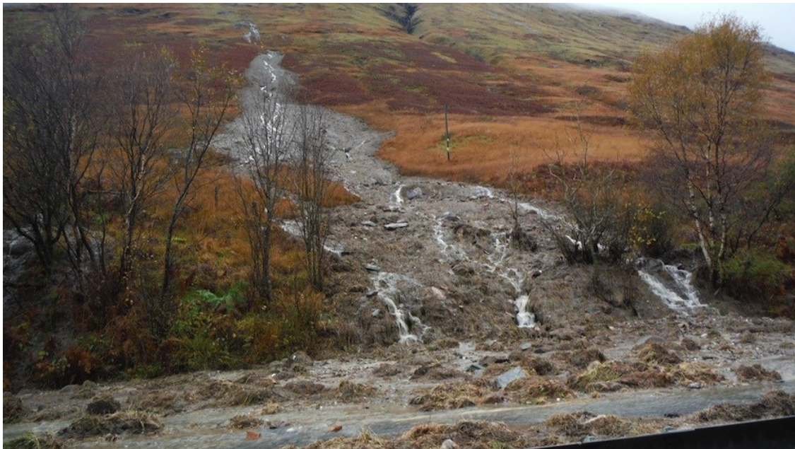
Figure 3.3. Debris flow on the A83 road near the Rest and Be Thankful pass 2014. Image taken from http://forargyll.com/?p=90101
