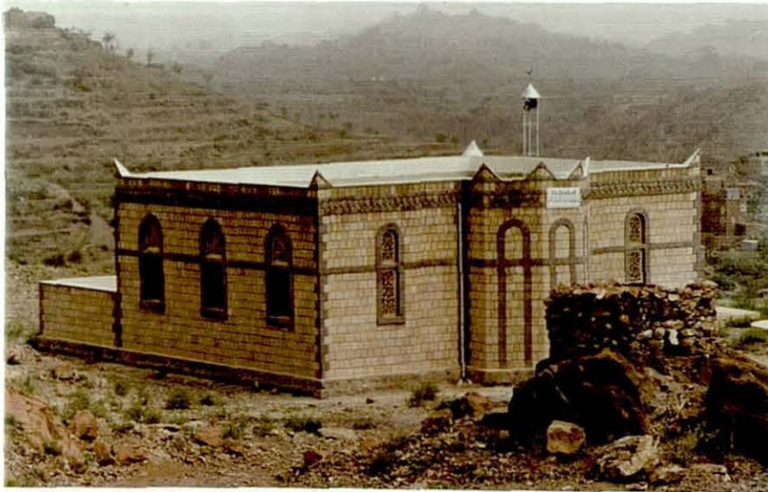
Figure 4.15: A mosque in Dhamar
