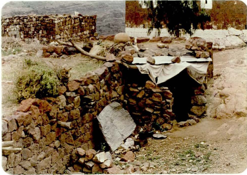
Figure 8.1: The non-beneficiaires still live in disaster prone houses Source: Field Surveys, 1994
